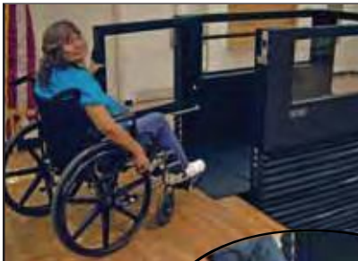
Dock plate facilitates easy stage-to-lift transition
