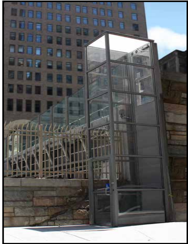
Morris Street Pedestrian Bridge, New York, NY
