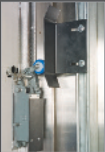
Car cam and roller position shut-off switch meet all industry codes as a dumbwaiter door safety interlock.
