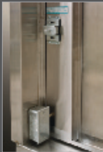
Key lock and door open shut-off switch meet all industry codes for a machine room access door interlock.
