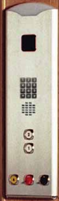
Inside operating controls (includes digital floor position indicator and integrated telephone)
